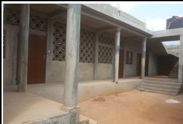
Drilling (black) on the top of the first floor of Sunday School building
